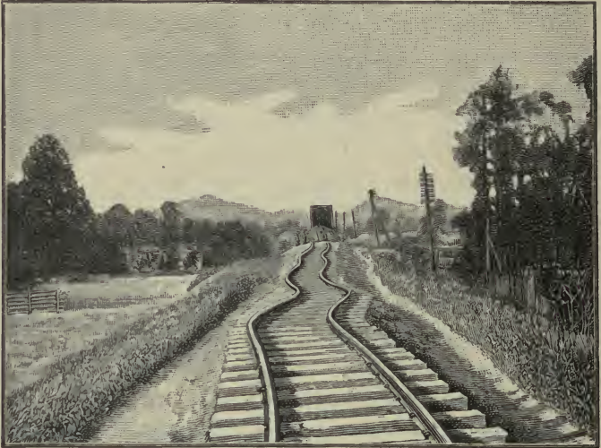
FIG. 97. Railroad shaken by an Earthquake, Northeastern India
